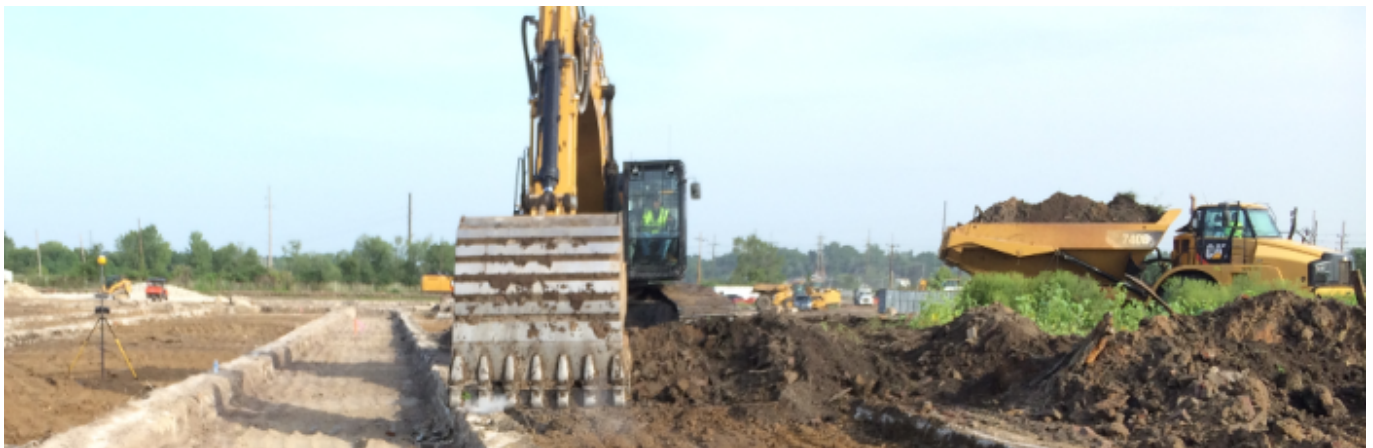
Figure 101. Final remedy in progress. Note GPS real time kinematic (RTK) base station on left side of photograph.
